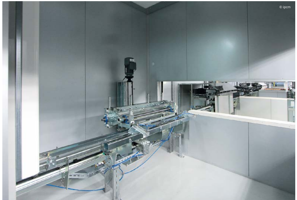
The second tilting station where the spindle is placed vertically before reaching the unloading area.
